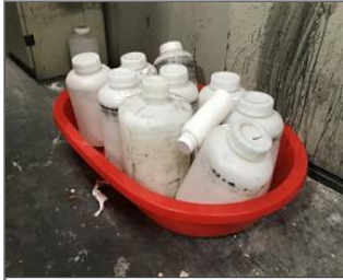
Photo of chemical storage room (if applicable) S4 Anti-leakage device for chemical.JPG
